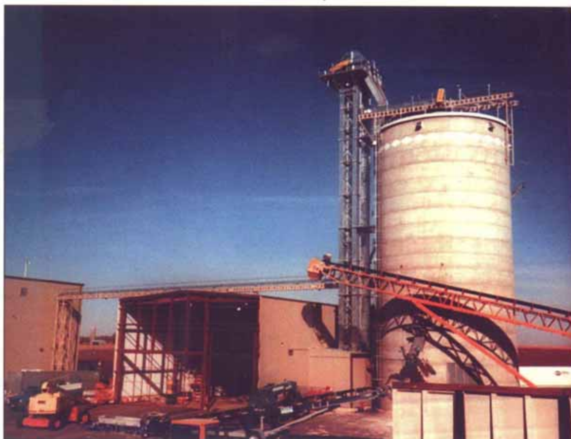
Siouxland Energy's new 14-million-gallon-per-year ethanol plant outside of Sioux Center, IA. Photos courtesy of Lambton Conveyor.
